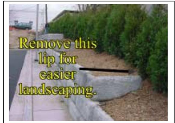
**B. Use the scalloped look:** Place Half-Top Blocks in a partial radius of 2 to 4 blocks to do this. Remove the outside knob on the last middle block of bottom course before beginning scallop. Simply make a few saw cuts through the knob and then hit it with a sledgehammer to remove knob (see middle picture at right).
